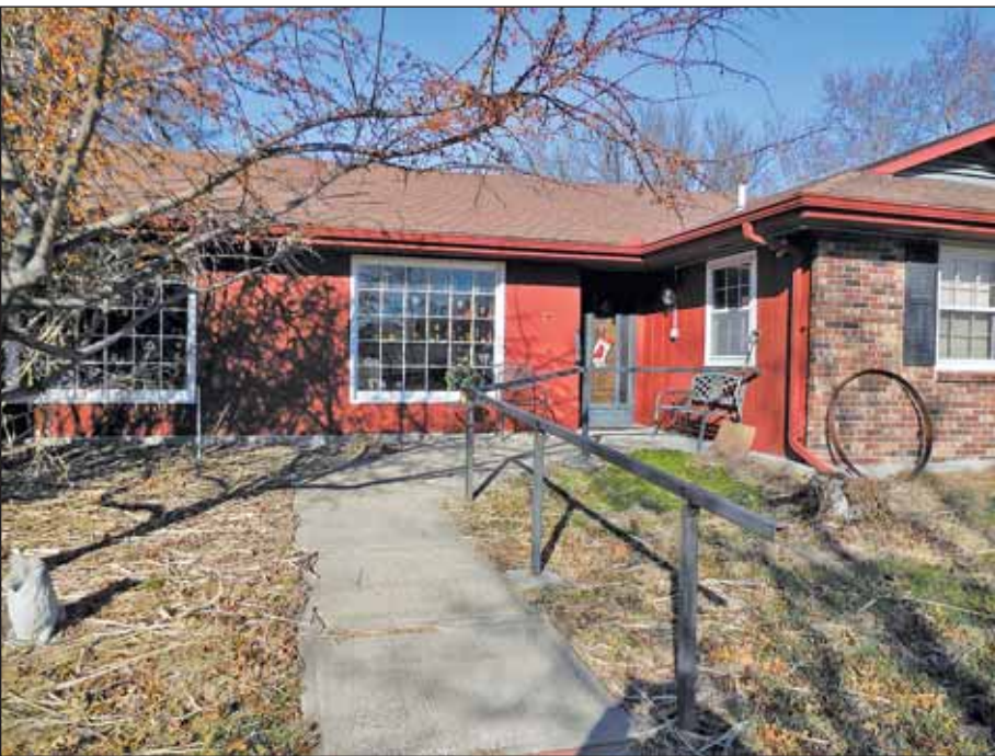
The gently rising sidewalk makes entering and exiting the house safe and easy.
