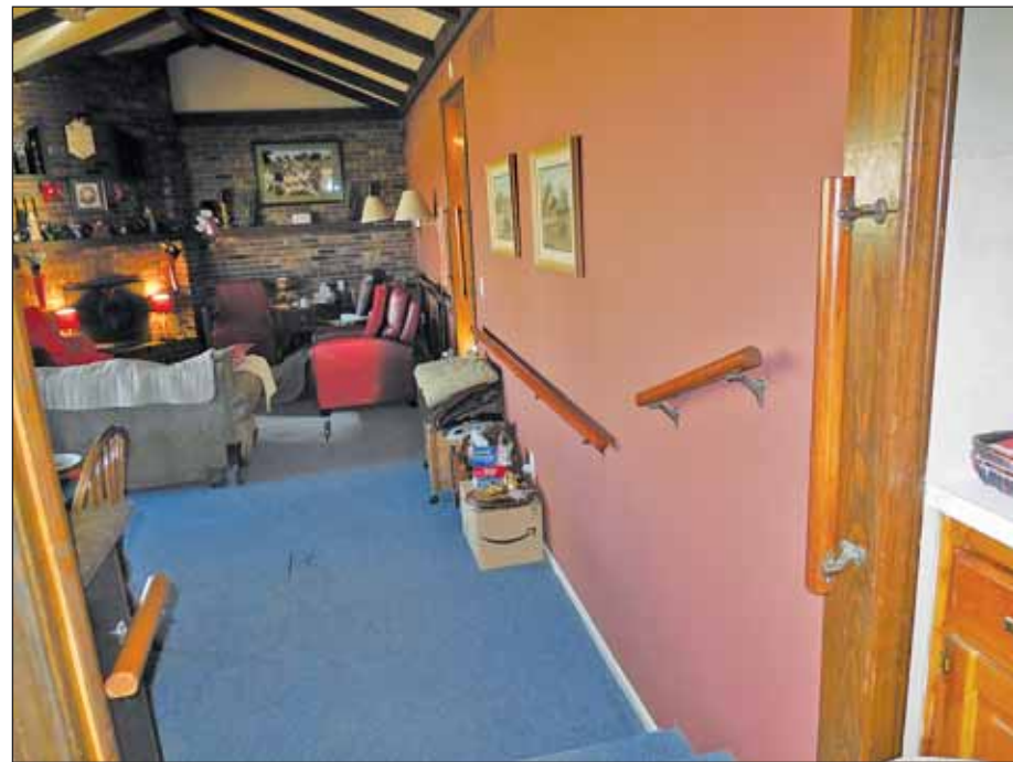
Grab bars and railings allow safe passage to the sunken family room from both kitchen and hallway.
